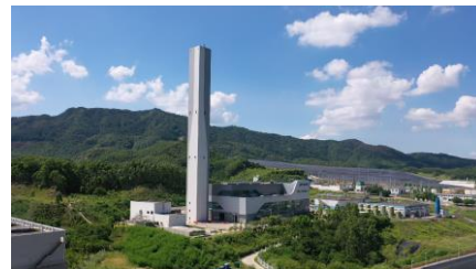
Foshan Medical Waste Treatment Project
